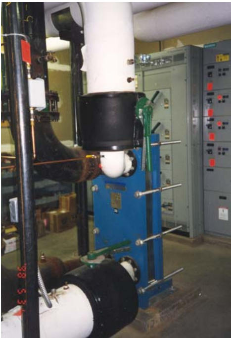
Figure 2. Photograph of one plate and frame heat exchanger at the Inn of the Seventh Mountain.
