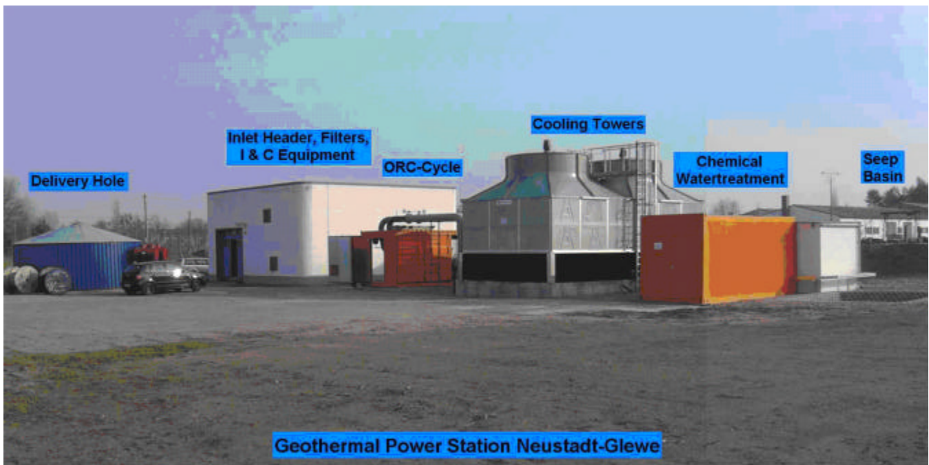
Figure 4. Entire geothermal power station.
