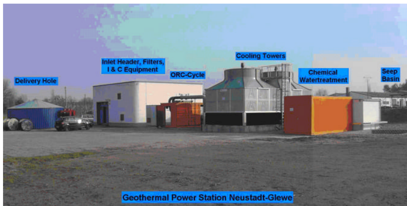
Figure 4. Entire geothermal power station.
