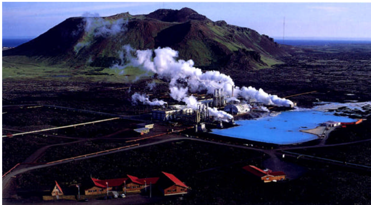
Figure 1. Svartsengi Power Plant aerial view.
