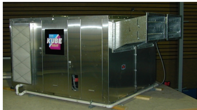
Figure 2. Dehumidification, air conditioning and heating are provided by a 20-ton heat pump in the ice area. The unit can cool and reheat 40-50°F (5-10°C) air. It can also cool or heat the arena by either rejecting or drawing heat from the horizontal earth loop.
