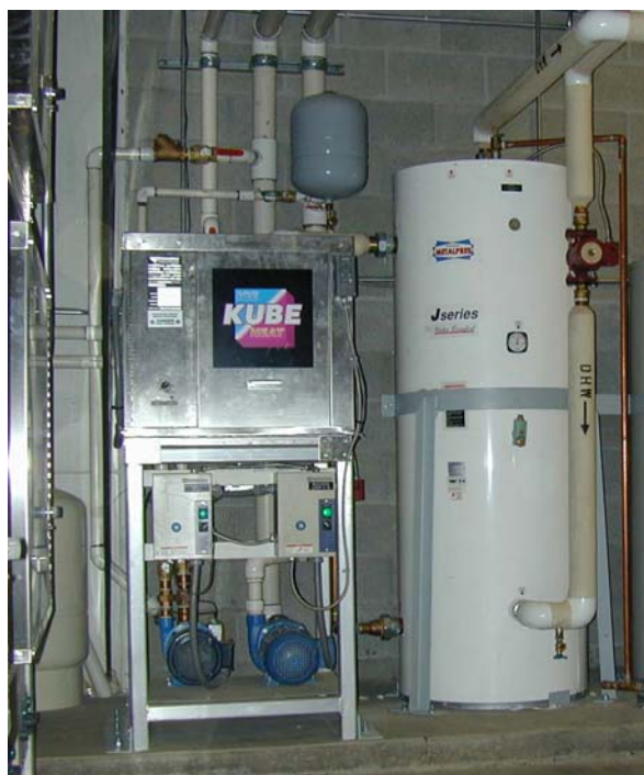
Figure 5. A 10-ton water-to-water heat pump draws heat from the earth loop to produce service hot water (showers and ice flooding) at 120°F (50°C)
