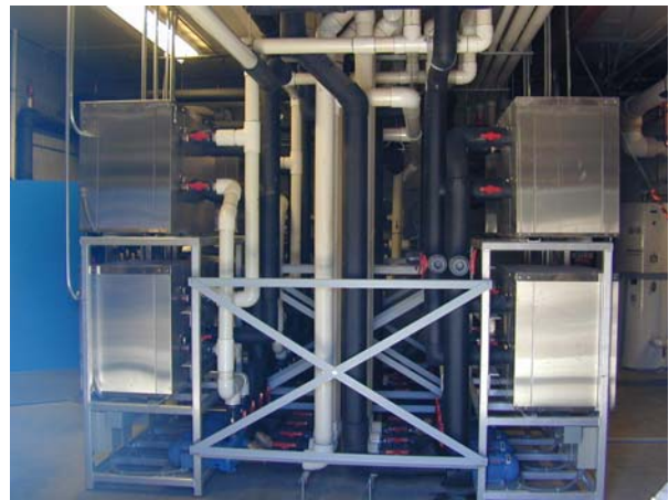
Figure 1. Eight low temperature water-to-water heat pumps provide approximately 84 tons of refrigeration at ice rink temperatures. The heat pumps reject heat either directly to a radiant floor heat system or to a horizontal earth loop.
