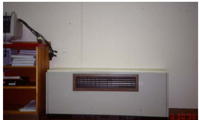
Figure 2. Console heat pump.
