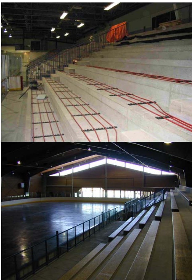
Figure 3. Much of the building, including the spectator seating, is heated with a radiant floor heat system. The warm floor dries snow that is tracked from outside into the building and reduces the opportunity for mildew growth in the change rooms.
