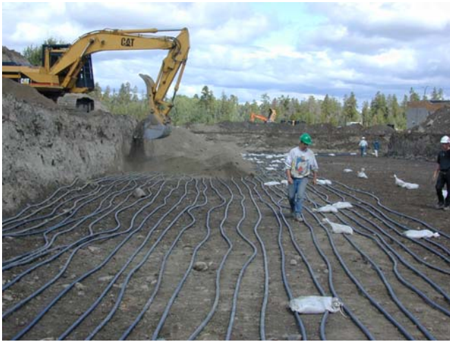
Figure 6. This photo shows the installation of the horizontal earth loop at 100 Mile House, BC. 50,000 feet (15,200 m) of 1 inch (25 mm) pipe was installed to a depth of 8 feet (2.4 m).
