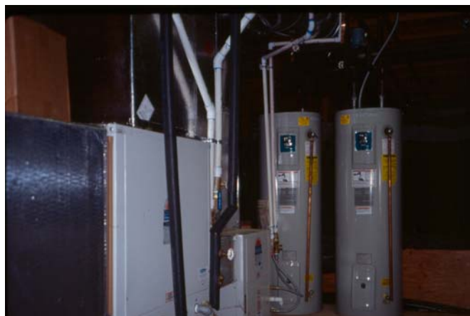
Figure 3. Water to water heat pump.
