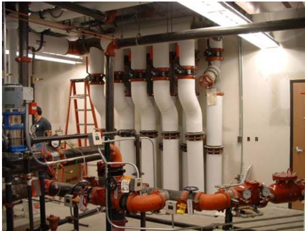
Figure 3. Photograph of the main mechanical room at the Murray High School, showing the ground loop field supply and return headers.
