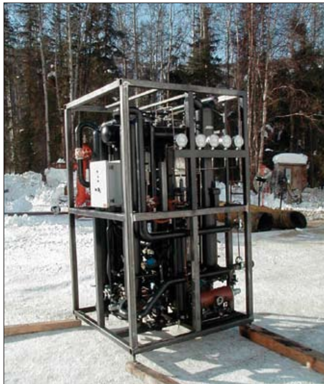
Absorption Chiller prior to installation.
