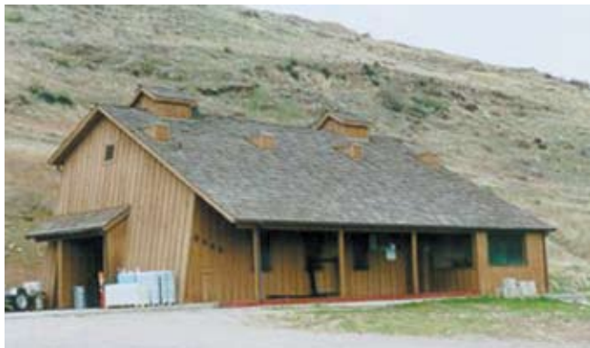
Warm Springs wellhouse
