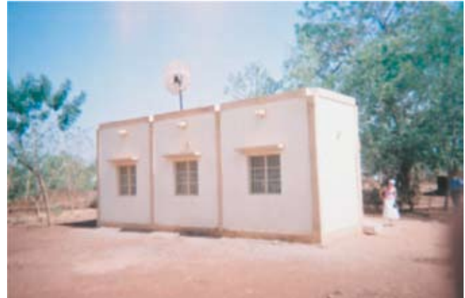
Figure 1. A typical building used in geothermal cooling experiment
