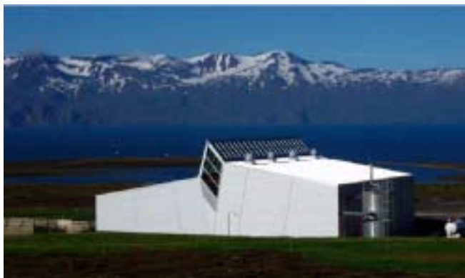
Figure 7: Husavik Kalina Binary Plant.
