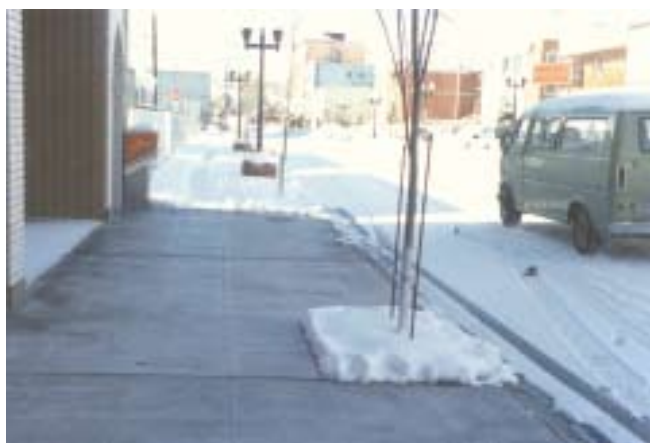
Photo 4: Geothermally Heated Sidewalk Snowmelt (Geo-Heat Center)
