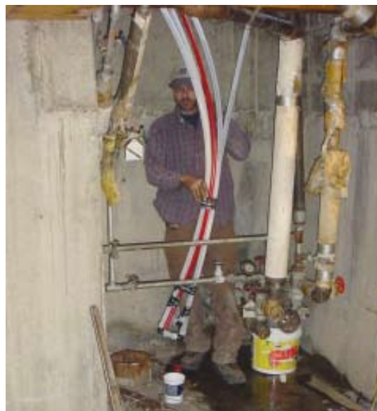
Figure 3. Photograph of double u-tube PEX DHE assembly prior to insertion into the well with dark (red) promoter pipe.
