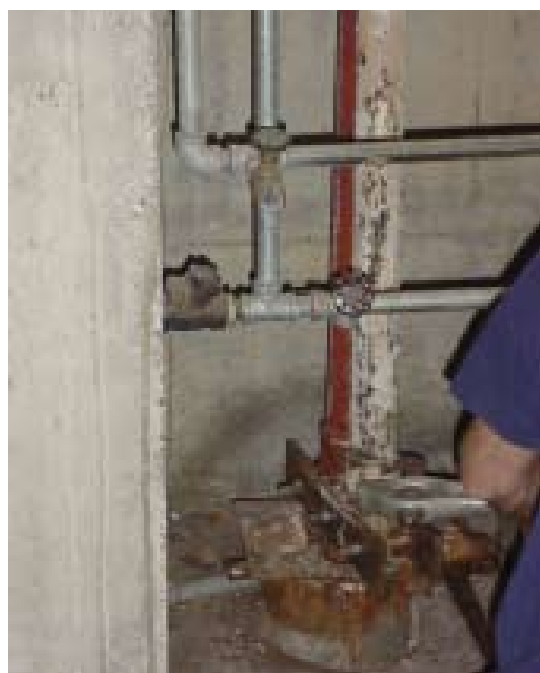
Figure 2. Photograph of removal of old black iron DHE, showing heavy scale deposits and corrosion.
