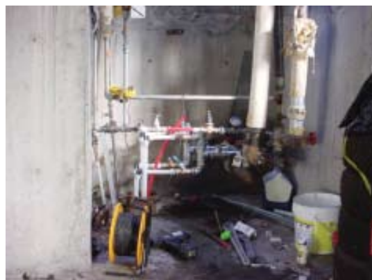
Figure 4. Photograph of the completed double u-tube PEX DHE.
