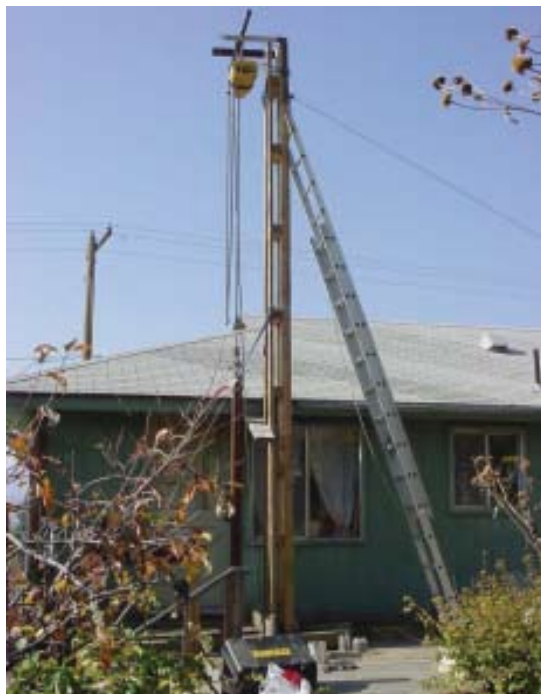
Figure 1. Photograph of removal of old black iron DHE.
