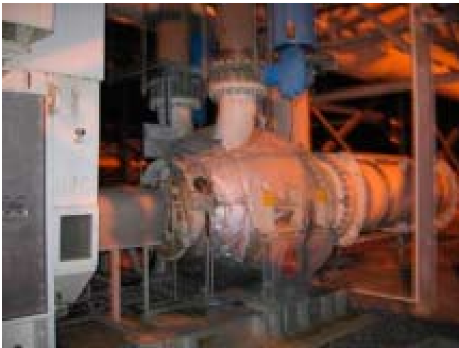
Figure 14: Salavatli Binary Plant.
