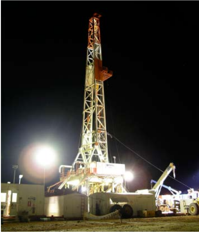
Figure 6. Drilling of Haanero I in the Coocer Basin (Geodynamics, Ltd.)
