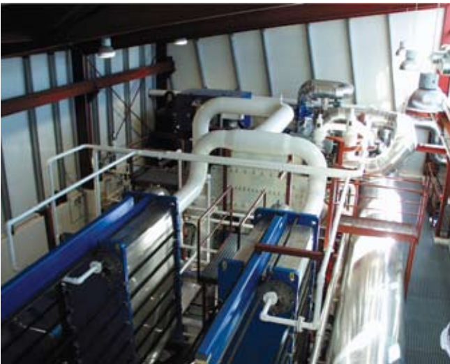
Geothermal power plant detail (exorka).
