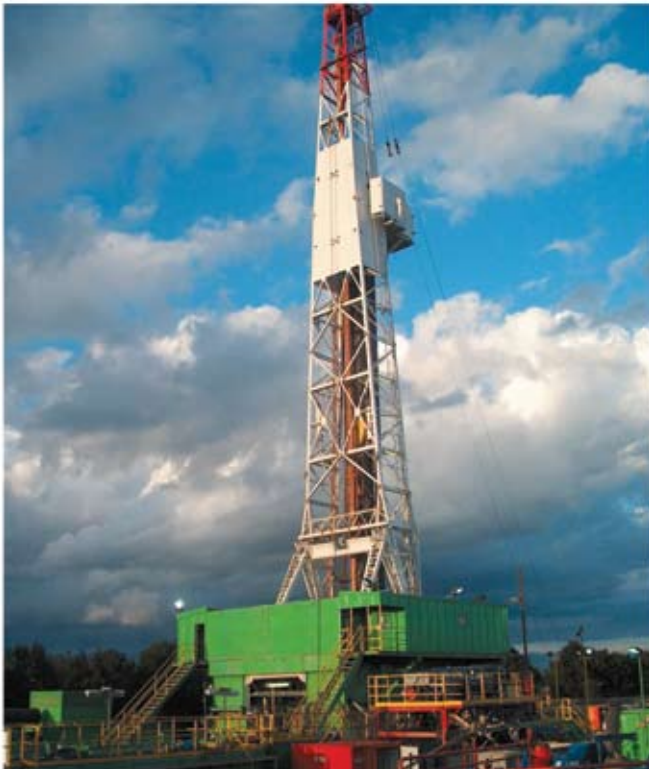
Derrick with 54m height for drilling the reinjection drill-hole. At the rear side one can see the assembled drilling rods with a length of 27m.
