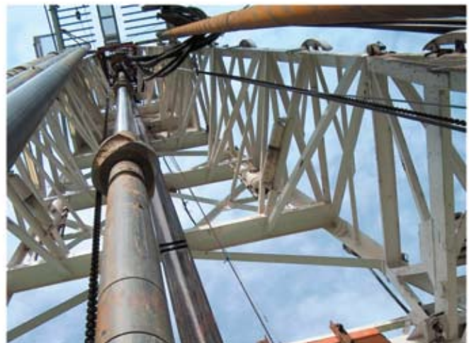
View upward to the top of the derrick along side the drilling rod. In order to gain time for the round trip three drilling rods of 9m each are assembled.
