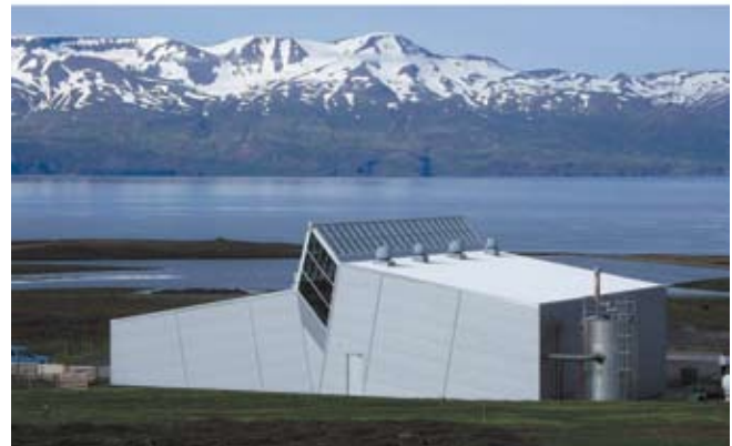
Geothermal power plant Husavik, Iceland (exorka).
