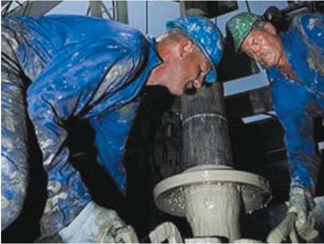
Disassembly of drilling rods after finishing a drilling tour.
