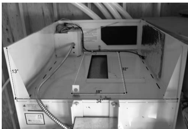
Figure 8: Target Size of New Opening
