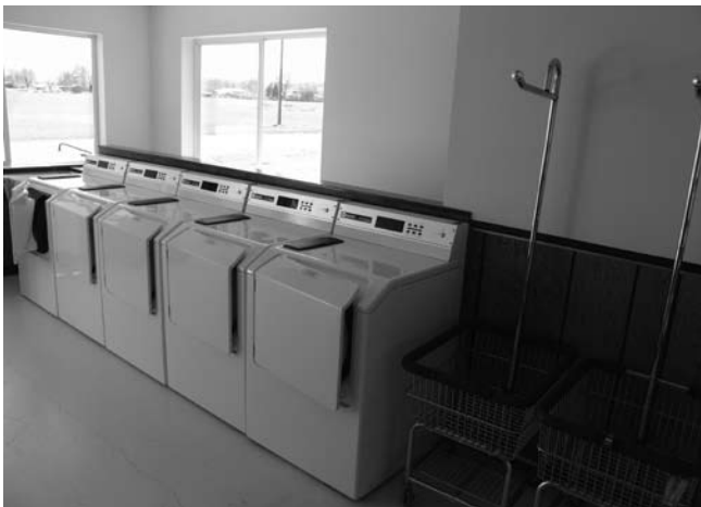
Figure 5: New High Efficiency 21 lb Washers
