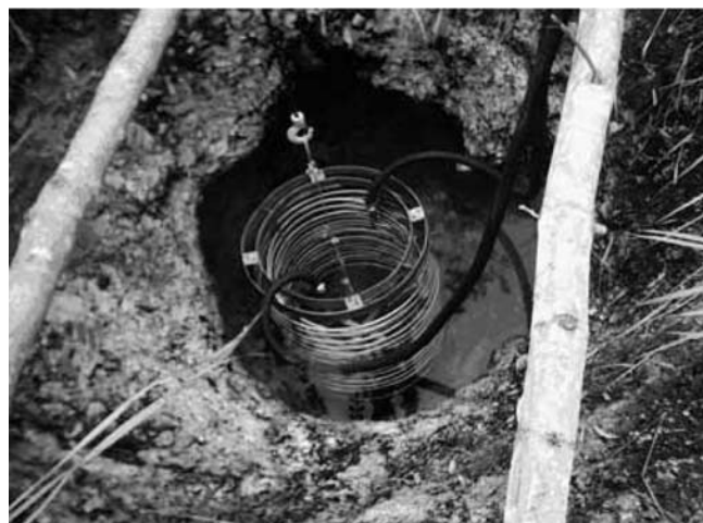
Figure 8: Downhole Heat Exchanger in Natural Geothermal Well
