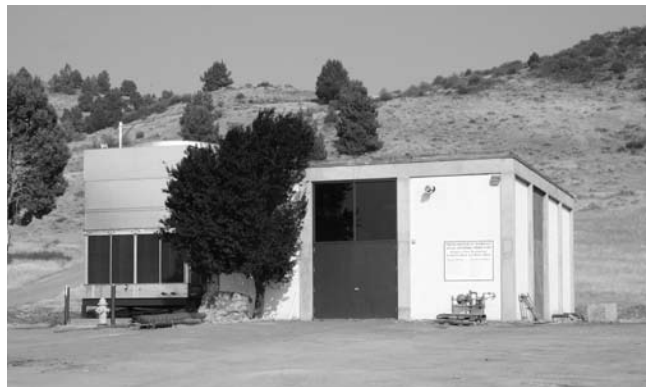
Figure 10. Building housing the low-temperature power plant and the associated cooling tower.
