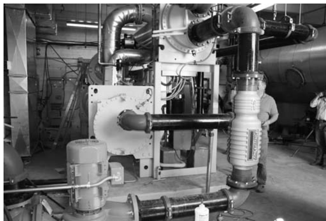
Figure 9. The low-temperature power plant inside the building.
