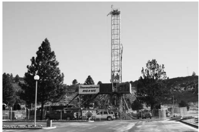
Figure 8: ThermaSource drilling rig on the OIT campus.
