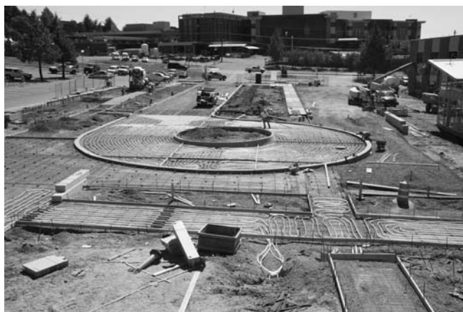
Figure 6: Installation of PEX pipe for the campus entrance snow melting system in 2008.
