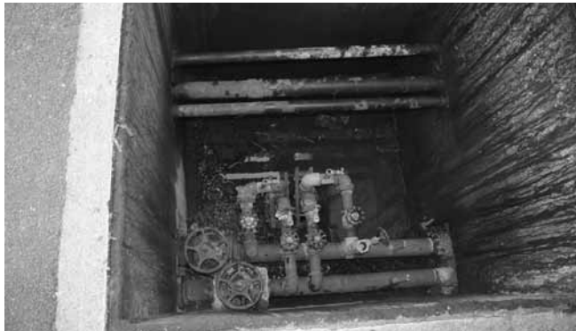
Figure 5. Roosevelt geothermal well with two 6.4-cm diameter downhole heat exchangers. The pipes in the upper part of the photo are connected to the second well.
