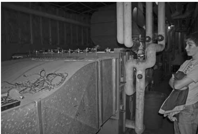
Figure 10. Finned tube heat exchangers supplying heated or chilled air to classrooms at Ponderosa Junior High School. Note the solenoid valves at the top of the heat exchanger that can be controlled to supply heated or chilled water.
