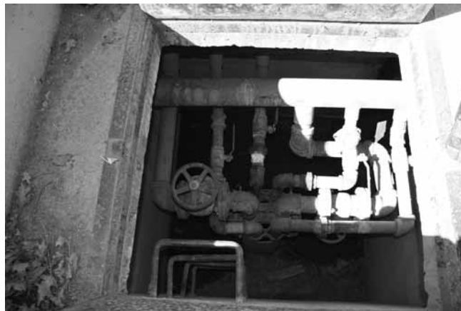
Figure 7. Downhole heat exchangers at Ponderosa Middle School: 2@5-cm and 1@ 7.5-cm diameter feeding into a common header.
