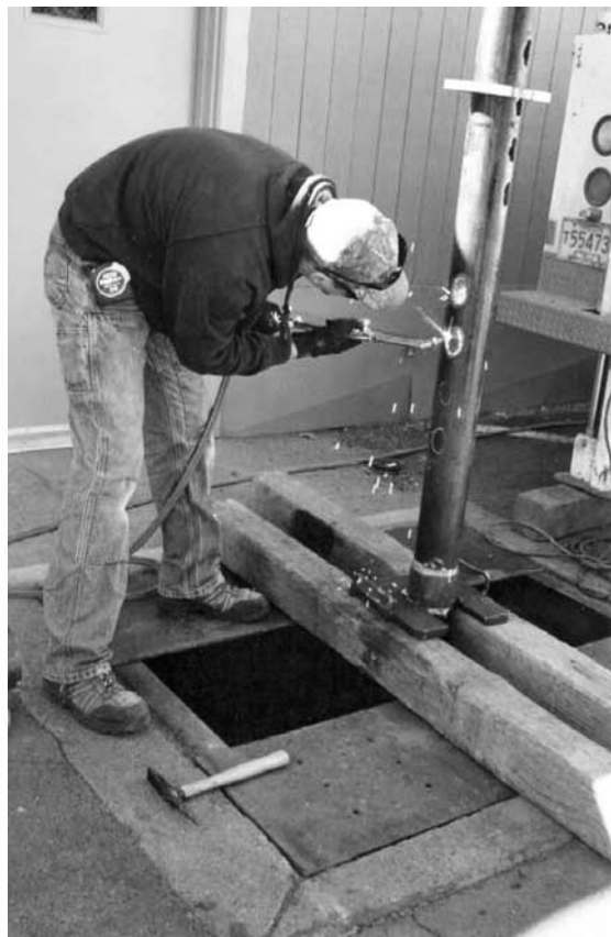
Figure 11: Cutting the 1-in diameter perforations in the promoter pipe for System Three.
