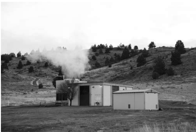
The power plant building with cooling tower.
