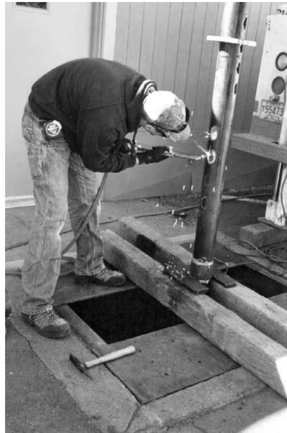
Figure 11: Cutting the 1-in diameter perforations in the promoter pipe for System Three.
