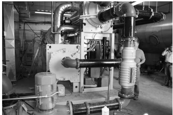
Figure 9. The low-temperature power plant inside the building.
