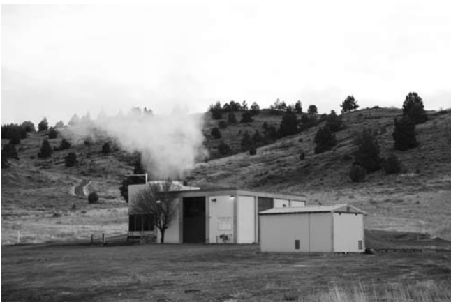
The power plant building with cooling tower.
