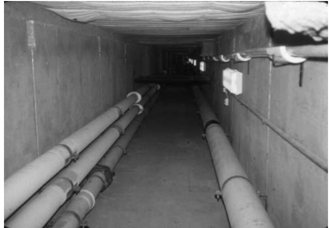
Figure 5: OIT utility tunnel with geothermal pipe and other utilities.
