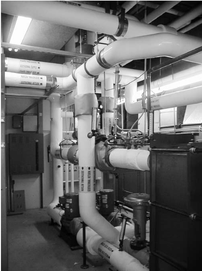
Figure 4: Plate heat exchanger in the College Union building.
