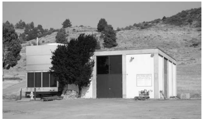
Figure 10. Building housing the low-temperature power plant and the associated cooling tower.
