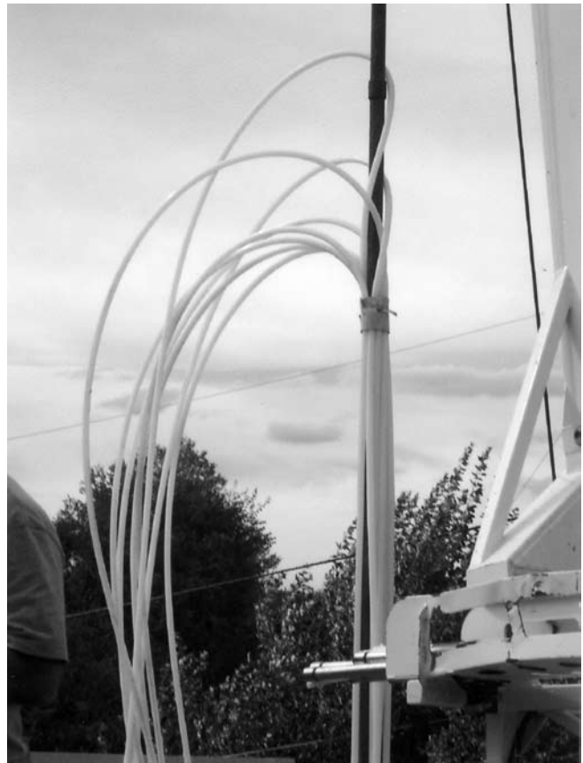
Figure 7: Placing the promoter pipe and PEX tubing into the System One well.
