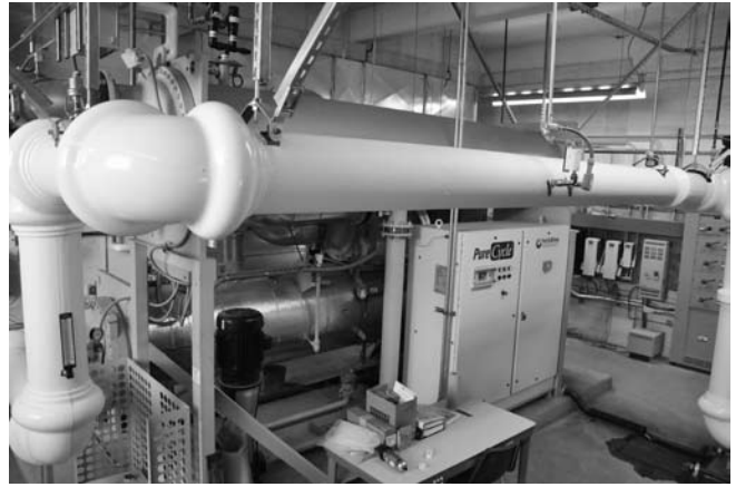
The power plant inside the building.
