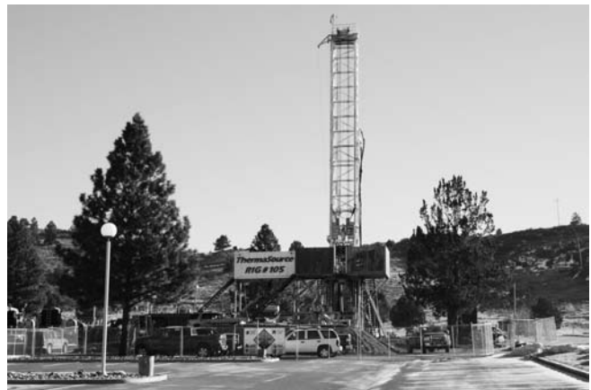
Figure 8: ThermaSource drilling rig on the OIT campus.
