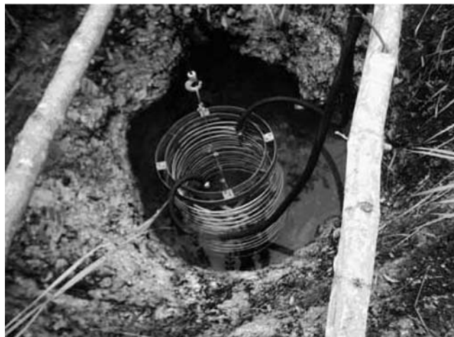
Figure 8: Downhole Heat Exchanger in Natural Geothermal Well
