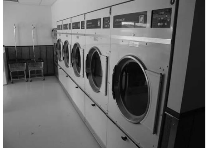
Figure 6: New Retrofitted 55 lb. Dryers
