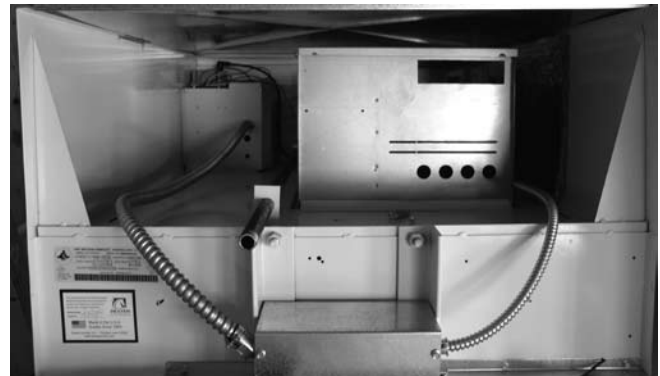
Figure 7: Gas dryer before retrofit
