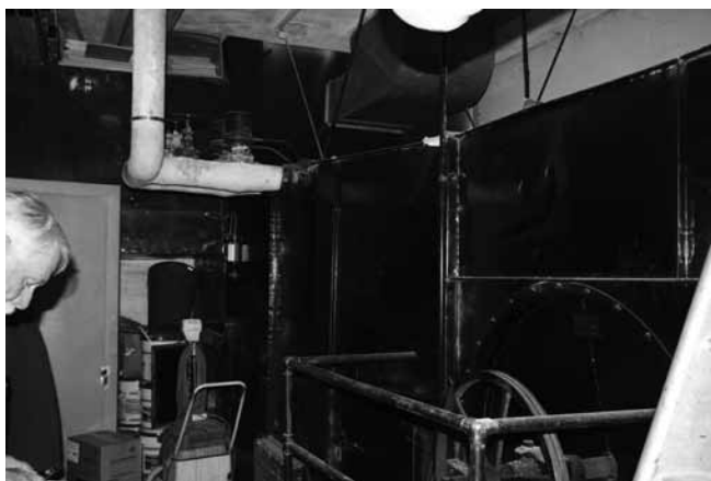
Figure 6. One of the two large force air units supplying heat air to the auditorium and supplemental heat to the classrooms.
