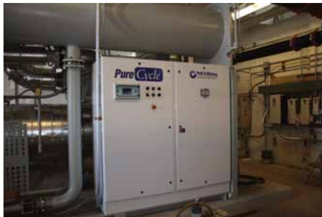
Fig. 4. The control panel for the 280 kW binary power plant.
