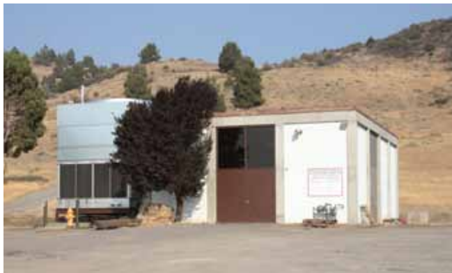
Fig. 5. The building on the OIT campus housing the 280 kW power plant, with the wet cooling tower on the left.
