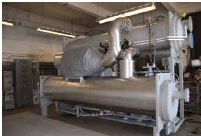
Fig. 3. The 280 kW binary power plant with the turbine-generator set (covered). The condenser shell-and-tube heat exchanger is on top and the evaporator on the bottom.
