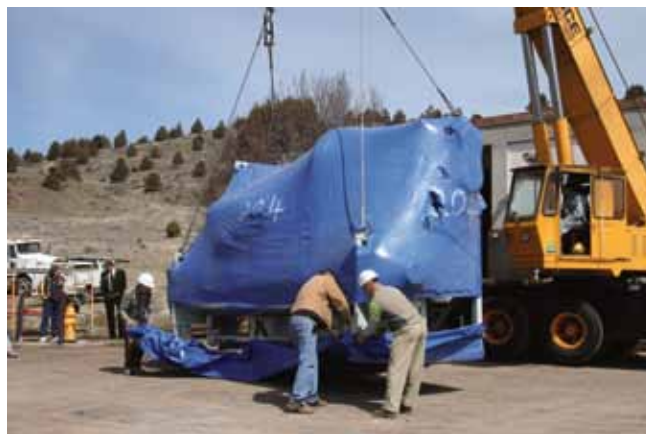
Fig. 2. Delivery of the UTC Pure Cycle© 280 kW binary power plant.
