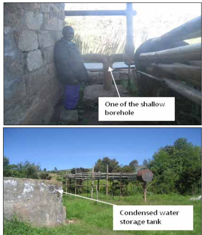
Figure 3. Shallow steam boreholes used for potable water and crop drying.
