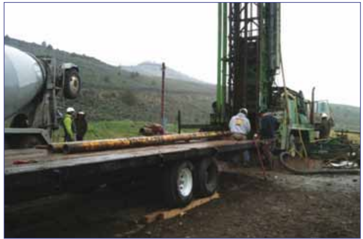
Figure 3. Paisley Drilling, May 2011.
