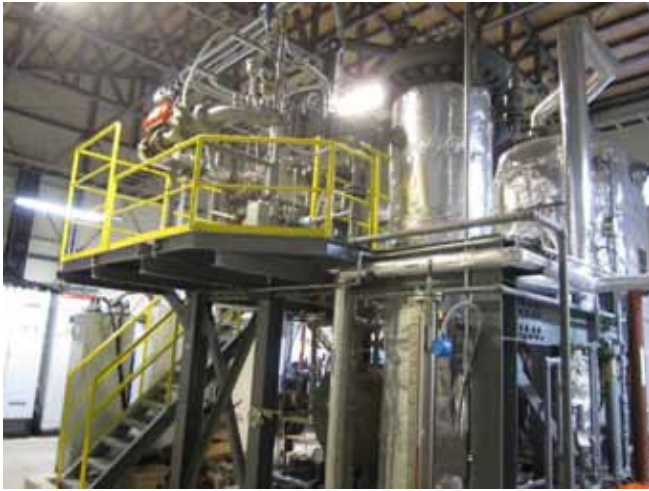
Figure 8. The Kalina power generation system using hot spring fluid at Matsunoyama.
