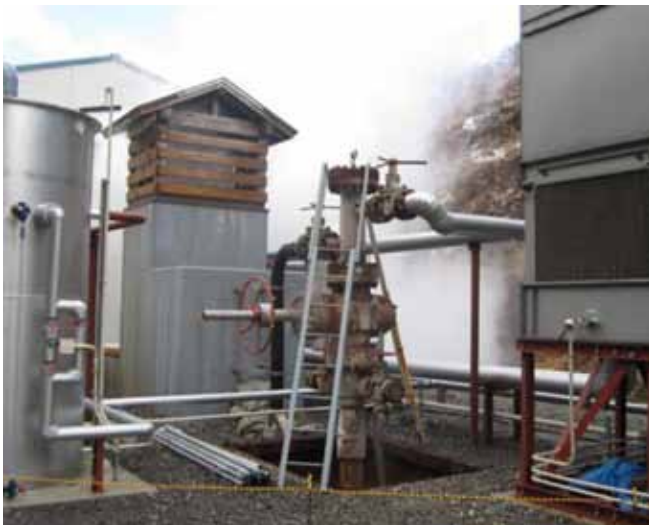
Figure 9. Wellhead of Takanoyu#3.
