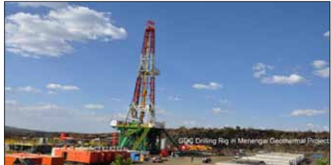
Figure 3. A GDC rig at Menengai Geothermal Prospect, GDC 2011.
