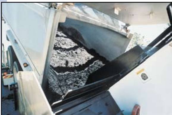
Even this mix can make a good pavement if it is run through a Roadtec MTV.
