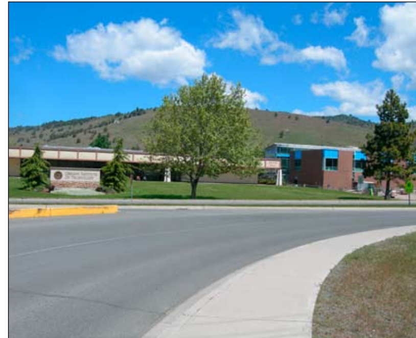
Entry 1. Extend stronger foundation plantings at the monument sign. Transplant cedar trees that will eventually crowd and shade the sign.
