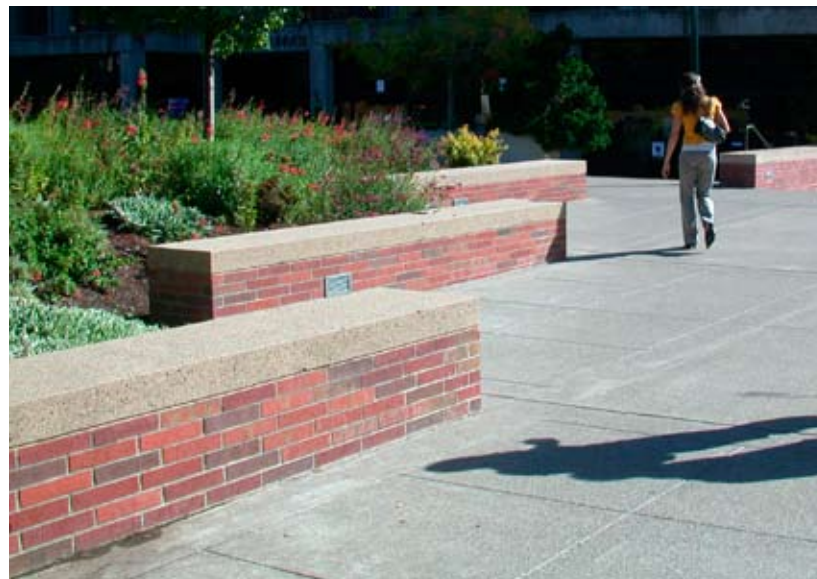
Low brick veneer retaining wall with precast concrete cap
