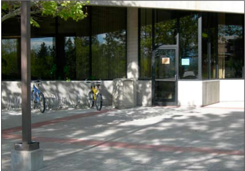
Replace temporary building signage with permanent campus standard signage.
