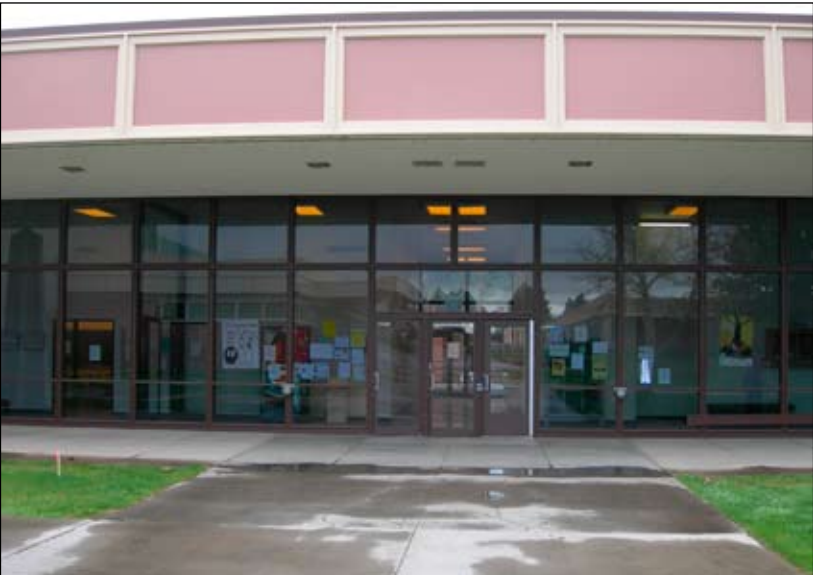
Provide a campus standard information board in foyer of building entrances to avoid the need for announcements taped to the glass.
