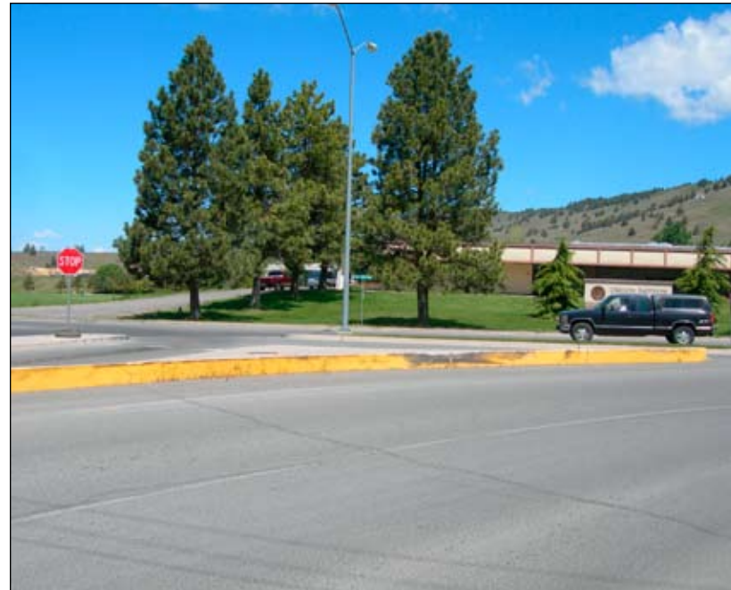
Entry 1. At the main campus entrance at Dan Obrien Way and Campus Drive, construct an inviting pedestrian walkway crosswalk and flashing traffic signal.
