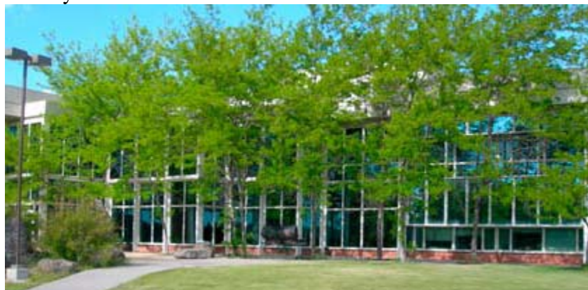
Figure 3. Deciduous trees planted at Purvine Hall reduce solar gain during the Summer, but allow for solar gain in the Winter (Mayer/Reed, 2007, p. 23).
